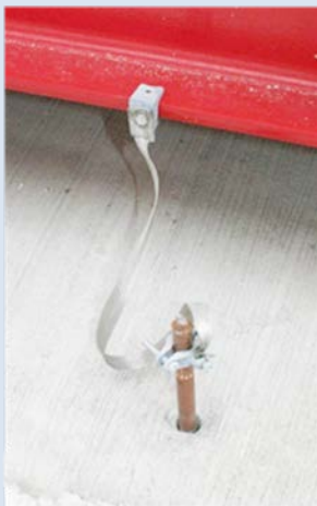
Proper grounding
